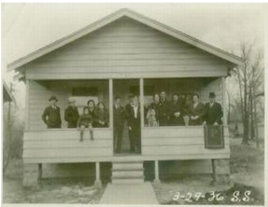
Figure 7. Becker cottage in Lake Como, Wisconsin.
